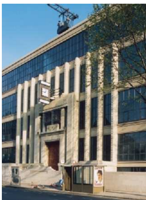
Figura 5 - Viyella House, Nottingham (Fonte DAWSONS (2003))
